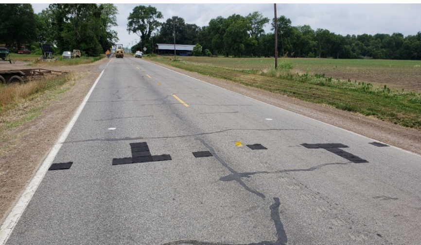
Geotextile pads placement on the test sections
