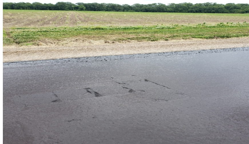
Geotextile pads after application of emulsion
